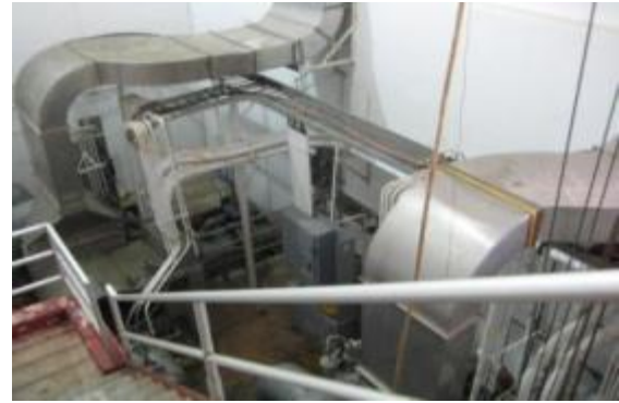
Figure 8: Hydro generators (Nanpil dam, Pohnpei)
