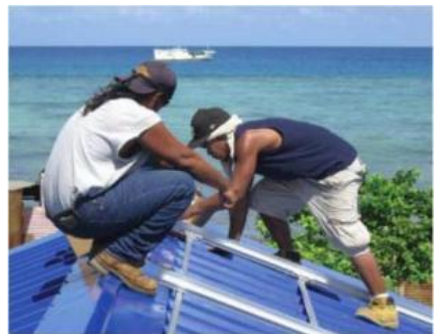
Figure 7: Installing solar module racks in the FSM. (source: Akker, 2006).
