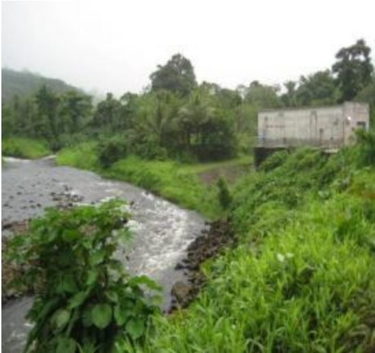
Figure 9: Hydro system in the Nanpil River, Pohnpei.
