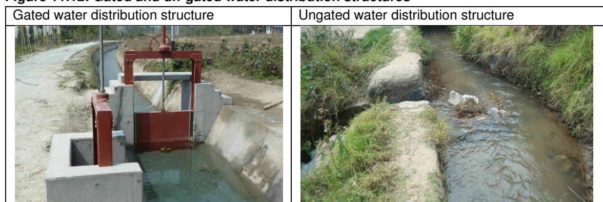
Figure 11.12: Gated and un-gated water distribution structures
