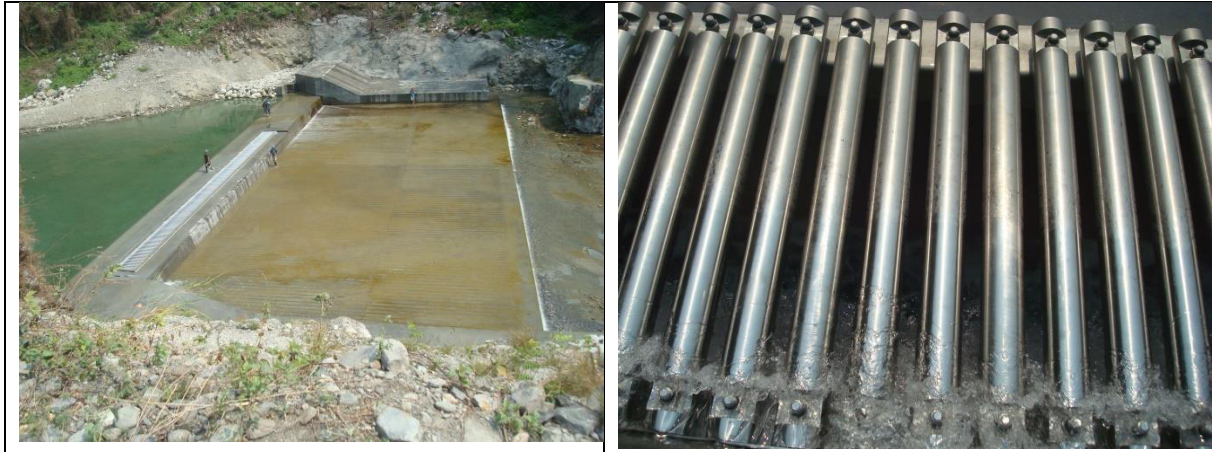
Source: ADB TA 8623 site visit
