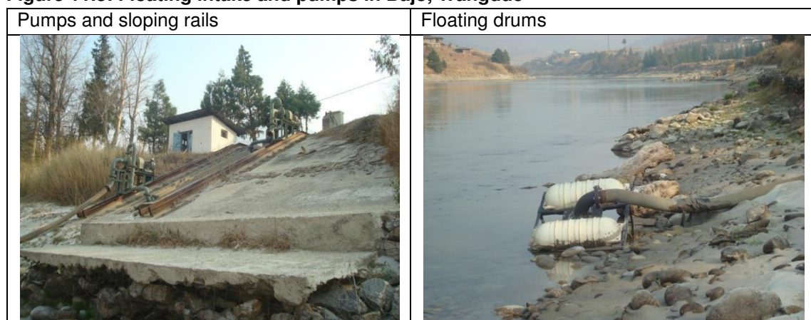
Figure 11.8: Floating intake and pumps in Bajo, Wangdue
