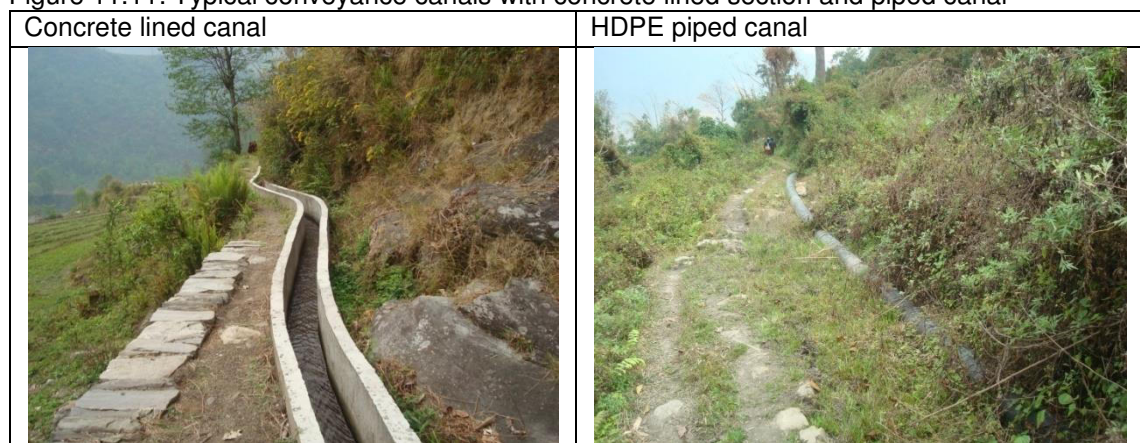
Figure 11.11: Typical conveyance canals with concrete lined section and piped canal
