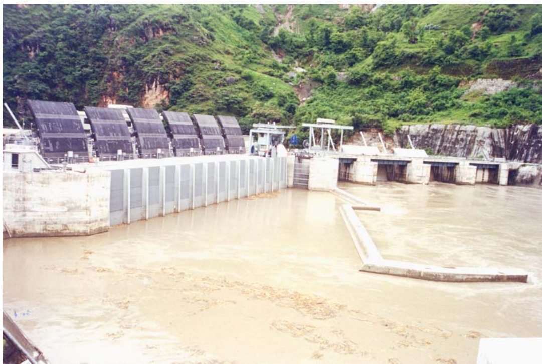
Plate 8: Upstream view of headworks, Kaligandaki Hydroelectric Project
