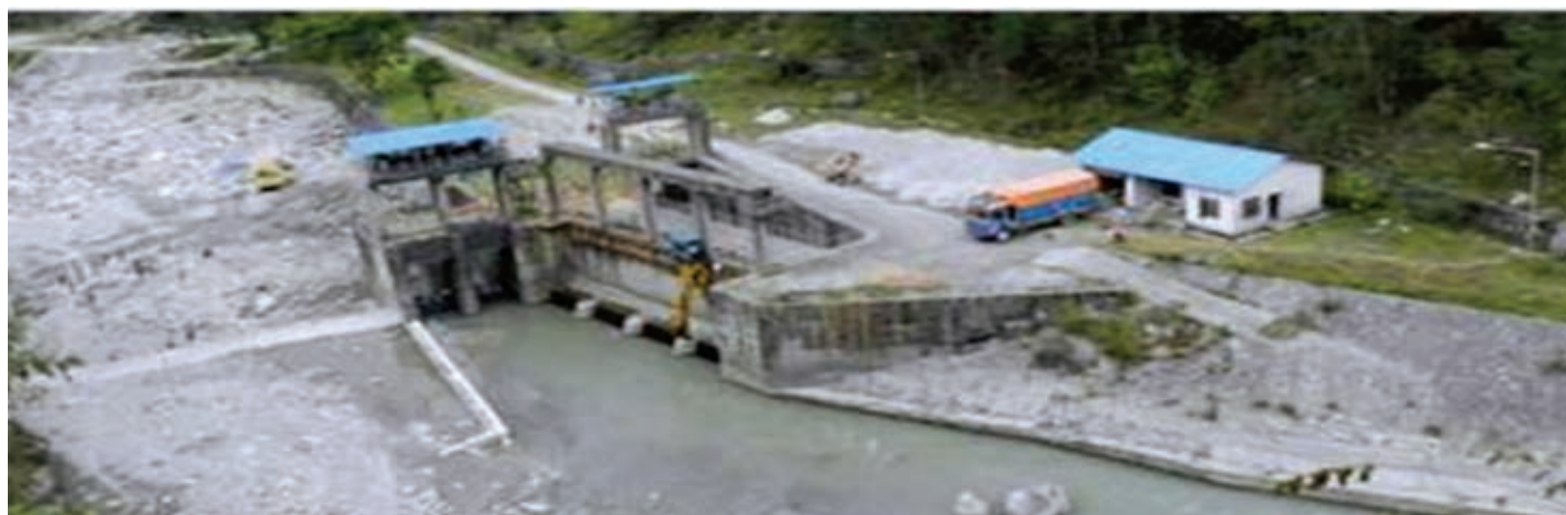
Hydro power station at Modikhola, Parbat district
