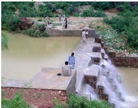
Delay action dam, Kaila, Soon Valley
