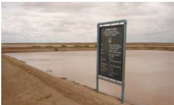
Rainwater harvesting pond--Khushkaba Bund, UC Jangian, Balochistan
