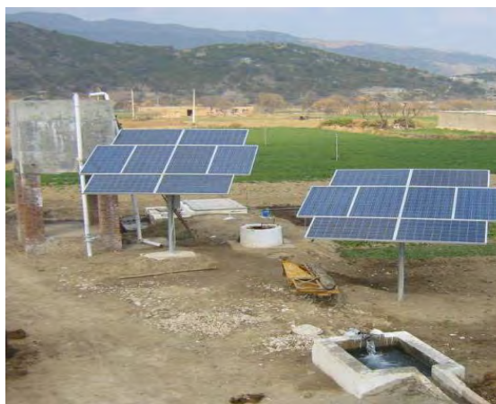
Solar powered irrigation system, Soon Valley, Khushab
