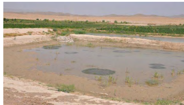
Rainwater harvesting pond, Pishin, Balochistan
