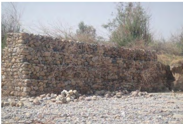
Flood protection wall
