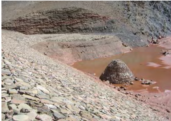
Delay action dam, Rodh Malazai, Balochistan
