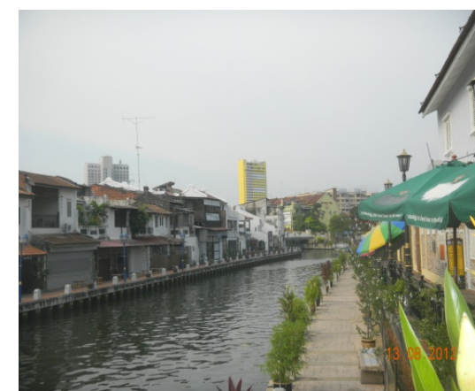
Retrofitting public buildings, Melaka
