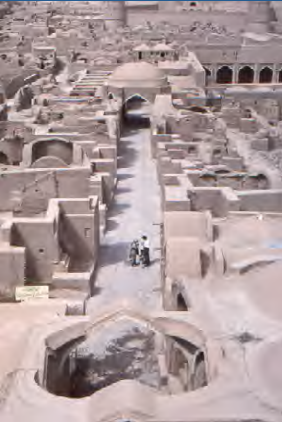
Bam-Iran: largest mud brick structures in the world, about 2000 years old. (WH in Danger)
